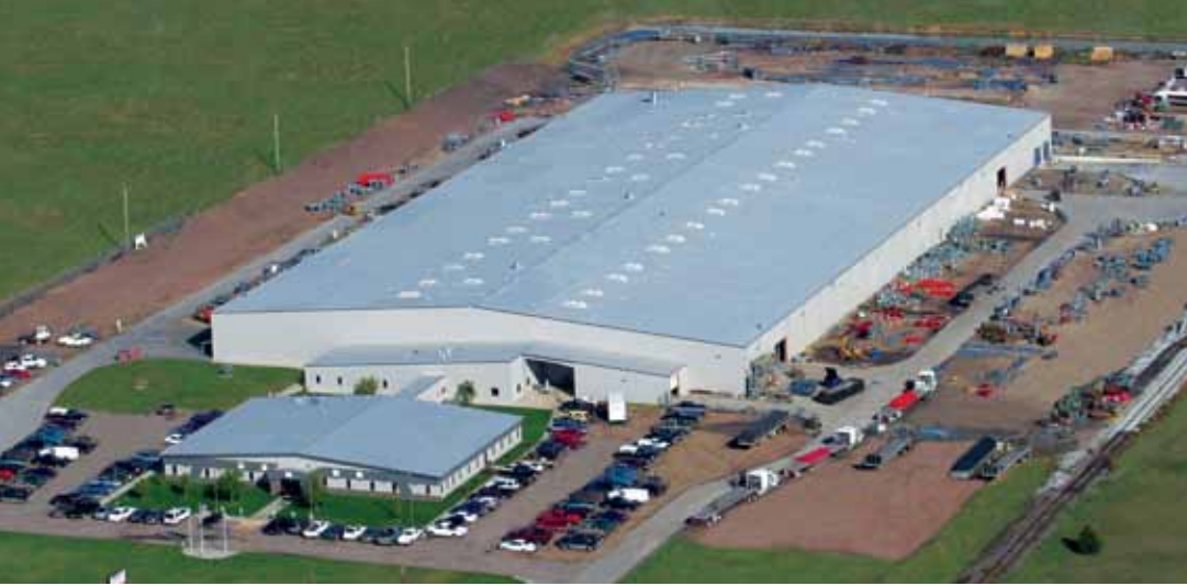
Aerial view of the Chief Agri/Industrial Division 178,640-sq.-ft. manufacturing plant in Kearney, NE. Photos courtesy of Chief Agri/Industrial Division.
