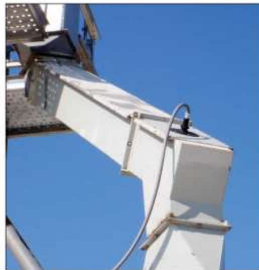
Binswitch Installed on Bucket Elevator Spouting (With SMP, BAS & A34NPT)
