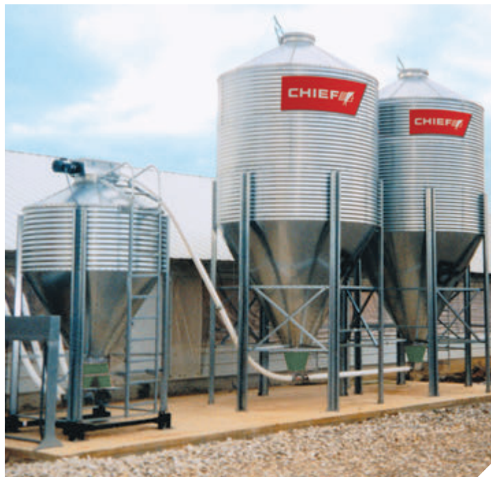
Chief flexible auger systems allow compact installations in a wide variety of configurations.
