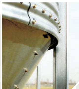
Drip edge directs moisture away from the taper hopper.
