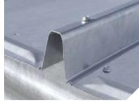
roof. Grain bins through 27'10" diameter have a 2½" depth. Bins from 30' 11" through 49' 6" diameter have a 4" rib depth. V-rib roofs are of the same G140 high quality galvanized steel as our commercial roof.
