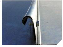
time. The structured "J" rib design gives the finished roof the strength it needs to support roof stairs and most conveyors.
