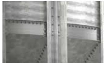
Built in compression ring installed on MDHT 5, 6, and 7 above 6 rings tall
